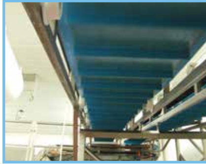
UHMW support on return
